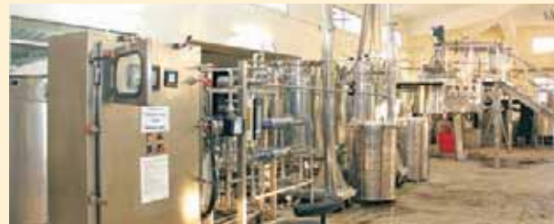
Pilot Plant for Developing Functional Food and Nutraceuticals
